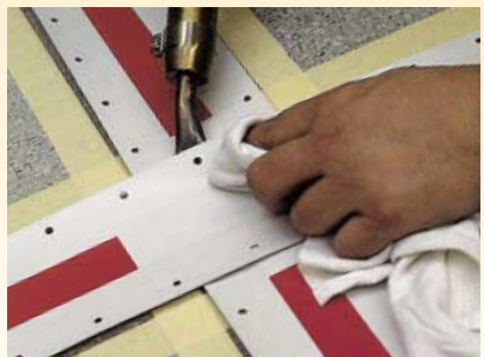
Hot air welding of joint details.
