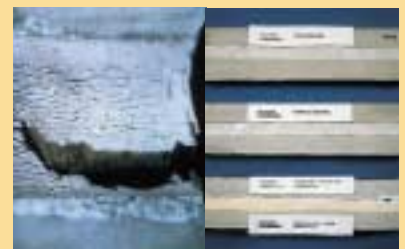
Conventional sealant after 3 month ozone exposure
