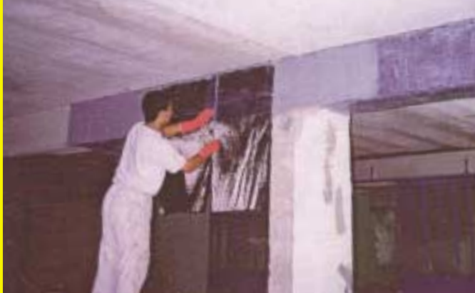
Shear strengthening of a beam in a building.
