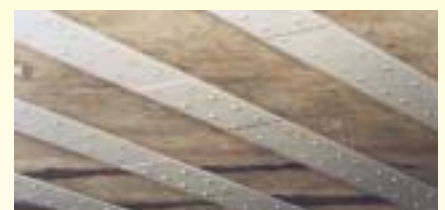
External steel plate structural strengthening with Sikadur® epoxy resin adhesive.
