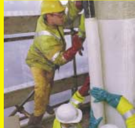
Impact strengthening of a bridge.
