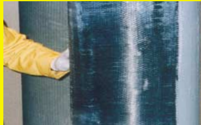
Strengthening for stiffness in a car park.
