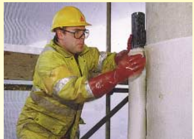
Application of SikaWrap® Fabric System for impact resistance on a bridge column.
