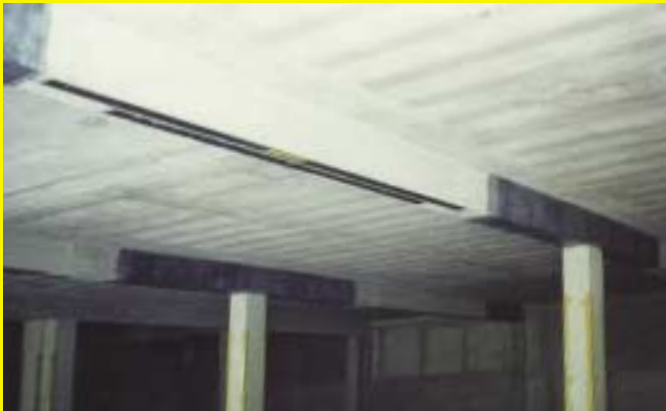
Shear and Flexural strengthening of a beam in a car park.
