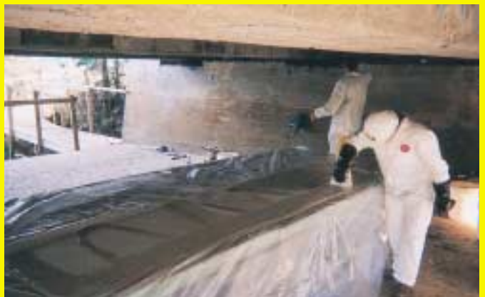
Shear strengthening of a bridge deck slab
