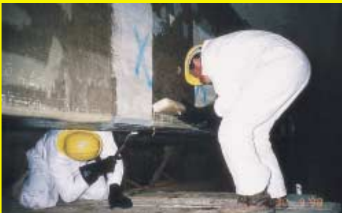
Shear strengthening of a bridge beam.
