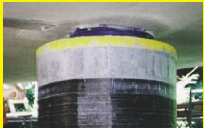
Restraint at the top of a bridge column.
