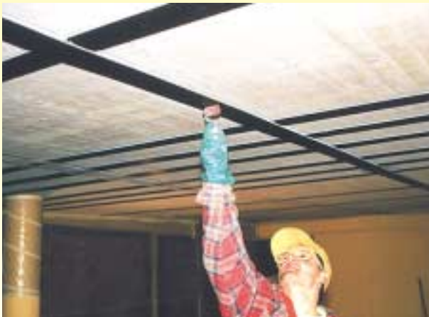
Strengthening of reinforced concrete slab with the Sika® CarboDur® Plate System.
