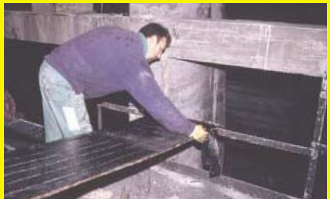
Shear strengthening of a slab in a car park.
