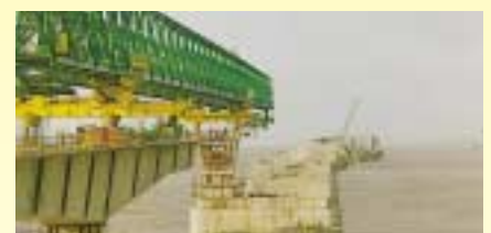
Segmental bridge construction with Sikadur® epoxy resin adhesive.
