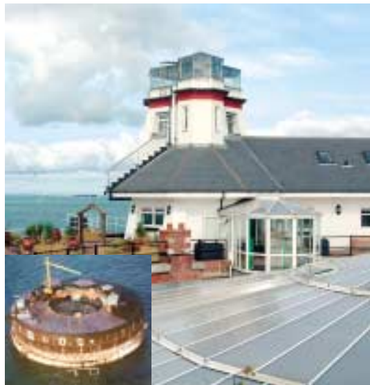
Weather joint sealing and elastic bonding to lighthouse building in the solent using Sikaflex® 11FC+
