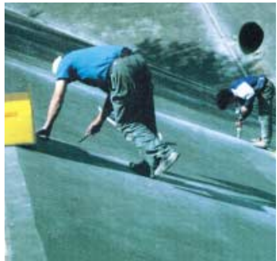
Chemical resistant sealing of sewage treatment works with Sikaflex® PRO-3WF
