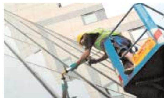
Sikaflex® PRO-2HP was used for resealing glass on this hotel
