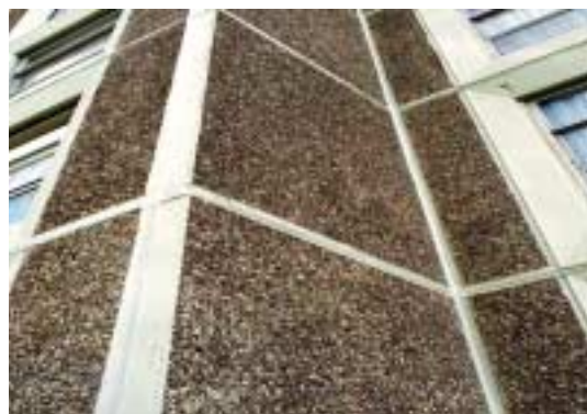
Sikaflex® PUR Band used on this residential structure to overband failed joints
