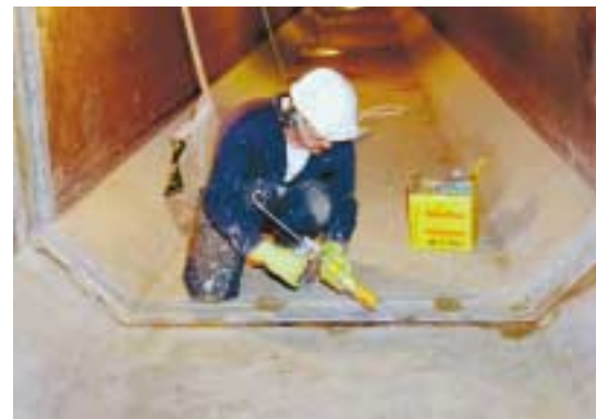
Sikaflex® 1A+ used for construction joint sealing in drinking water culvert
