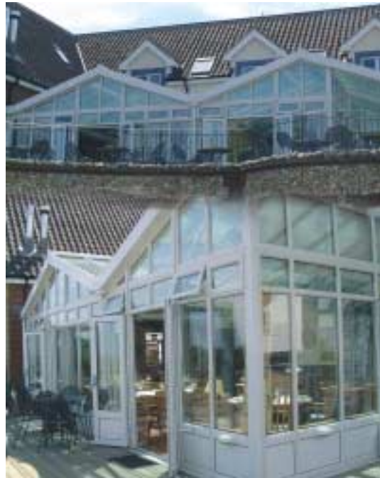
Perimeter sealing on conservatories with Sikaflex® Windowseal (photograph courtesy of N&P windows Hitchin)
