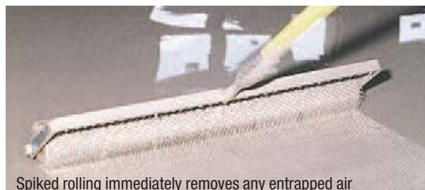
Spiked rolling immediately removes any entrapped air
