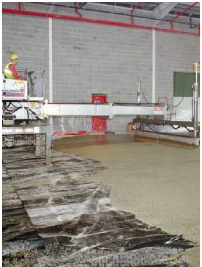
Laser Levelling Concrete
