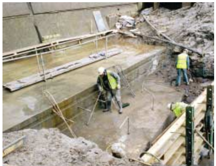
Stripping formwork and cleaning
