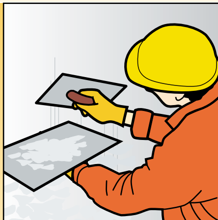
17. Final plaster finishes suitable for decoration can be produced with SikaMur® Finish .
