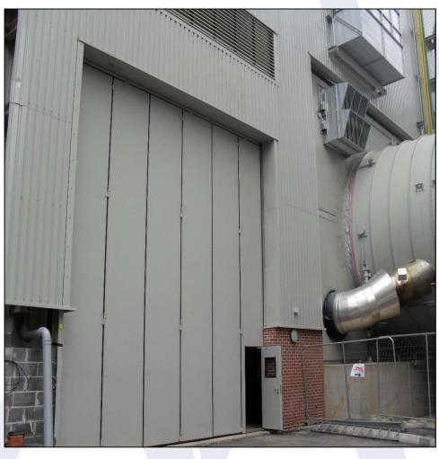
buttons adjacent to the opening at the bunch side. Disconnection for emergency manual operation is provided at low level at the motor side. Safety edges are fitted as standard to the leading edges.
