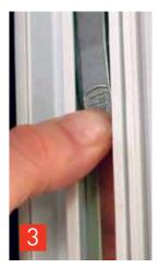
Once the safety catch is released the window can be completely rotated
