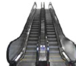
Escalators and moving walkways
