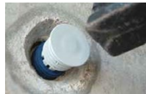
Hammer the TT Sealing Plug into the formwork spacer
