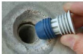
Position the TT Sealing Plug in the formwork spacer
