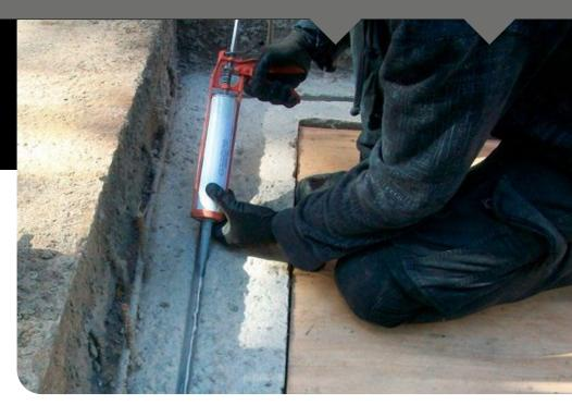
**TT Swellmastic S2** is a grey, elastomeric, swellable system which is applied into a pre-formed rebate within the concrete construction joint or when used with **TT Waterstop**. **TT Swellmastic S2** swells when it comes into contact with moisture. preventing passage of water through concrete construction joints.
