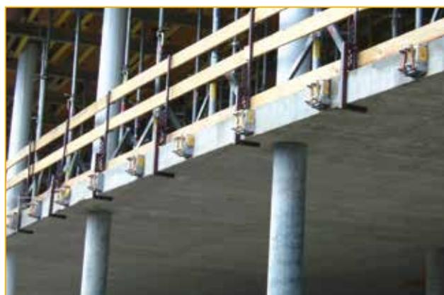
Figure 20: Schöck Isokorb® type KS incorporated into the interior slab. Steel balcony to be installed afterwards.
