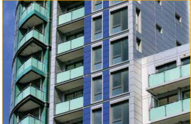
Figure 12b: Typical residential building, supporting structure made of concrete. Concrete balconies are thermally broken by Schöck Isokorb® type K.
