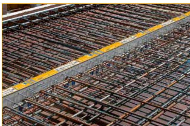
Figure 15: Schöck Isokorb® type K incorporated between the exterior balcony and the interior slab.
