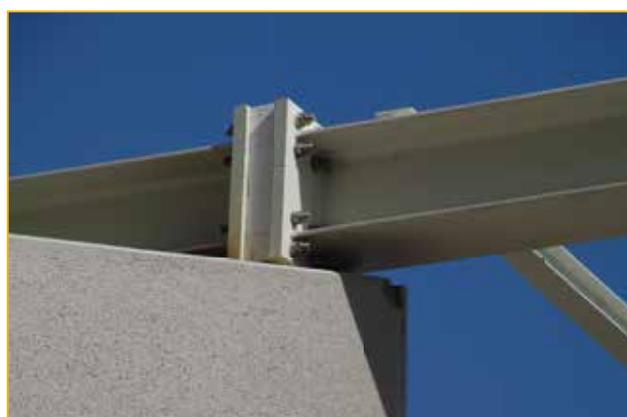
Figure 25: Schöck Isokorb type KST installed between the interior and the exterior beam.
