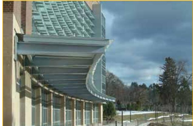
Figure 22: Typical building with supporting structure made of steel. Steel canopies are thermally broken by Schöck Isokorb® type KST.
