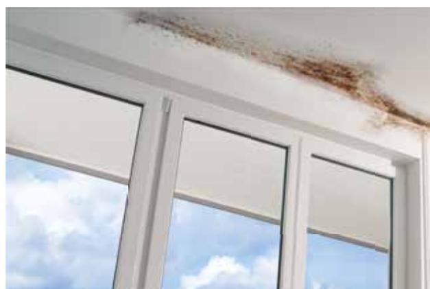
Figure 6: Photograph showing mould growth on the ceiling of a concrete slab adjacent to an exposed slab edge thermal bridge. Condensation forms here frequently as a result of colder interior surface temperatures.
