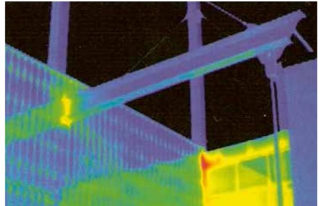
Figure 10: Structural thermal bridging in steel structures.
