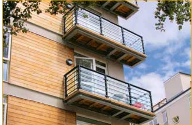
Figure 17: Typical residential building, supporting structure made of concrete. Steel balconies are thermally broken by Schöck Isokorb® type KS.
