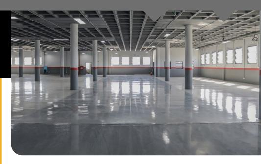
A solvent free, two-part epoxy resin coating primarily for use on screeded or concrete floors subject to rising damp or containing residual construction moisture.
