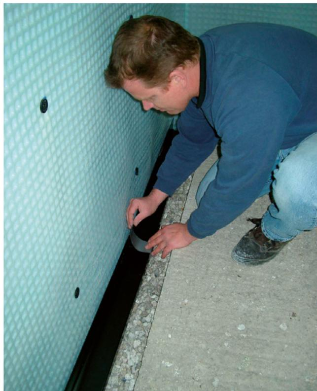
Fig. 21 Infilling to AquaChannel and gully with aggregate
