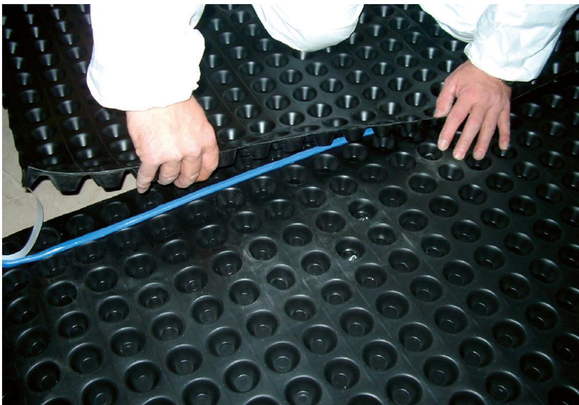
Fig. 8 Pressing membranes together to ensure bond
