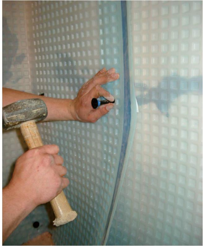
Figs. 3 and 4 Flange to stud Sealing Tape joint
