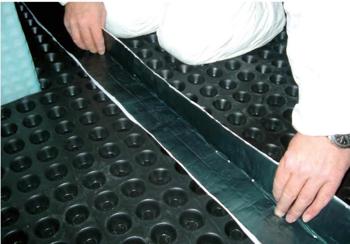
Fig. 10 Cornerstrip with crease offered into angle
