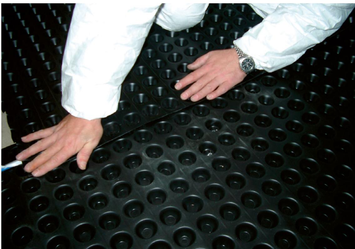
Fig. 9 Forming 90° angle crease in Cornerstrip
