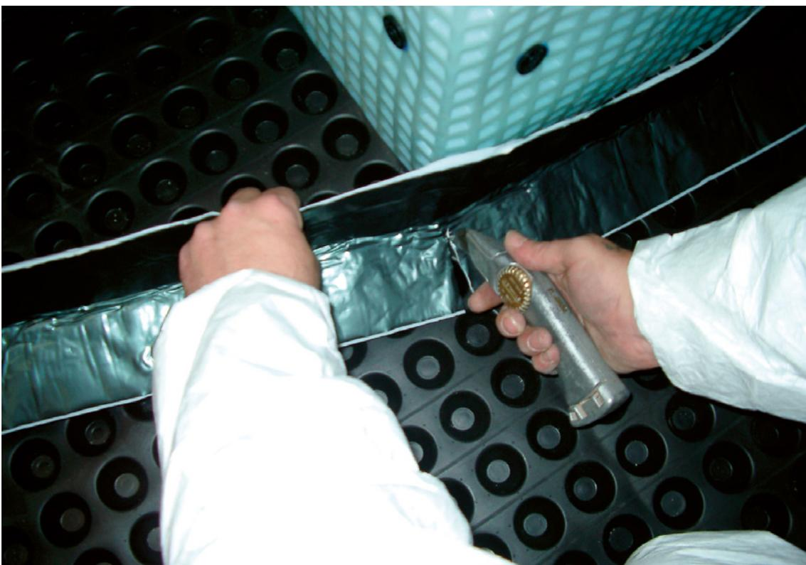
Fig. 12 Cornerstrip pressed into position
