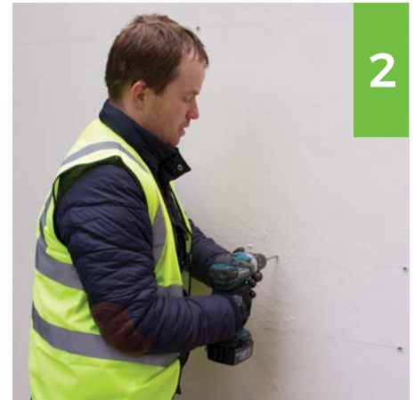
Drill the holes
