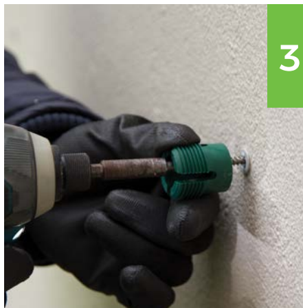
Plug & screw the fixing
