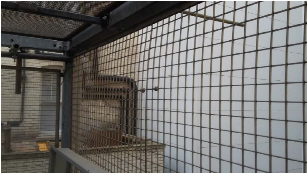
Metal cage before Vistafolia® installation
