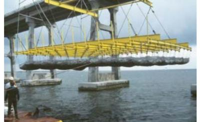
"We can select from a range of woven or non-woven geotextiles to suit the technical requirements; in the **Venice MOSE Project**, we even developed a specific **BFM** and deployment methodology to suit the project, combining engineering knowledge with manufacturing capability."
