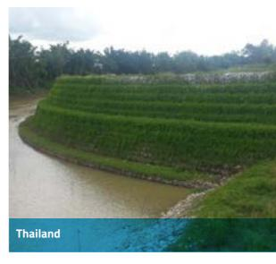
Revetments are suitable where the slope has localised shallow surface failures which do not affect the global stability.
