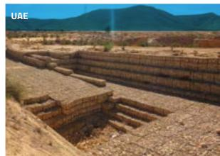
These grade control structures limit hydraulic erosion in the watercourse by reducing the hydraulic gradient and hence the velocity of the water to a value at which it ceases to dislodge soil particles in the river bed and banks.
