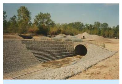
Gabions and Terramesh® are often used as the culvert headwalls and car be designed to support roadways or other infrastructure above"
