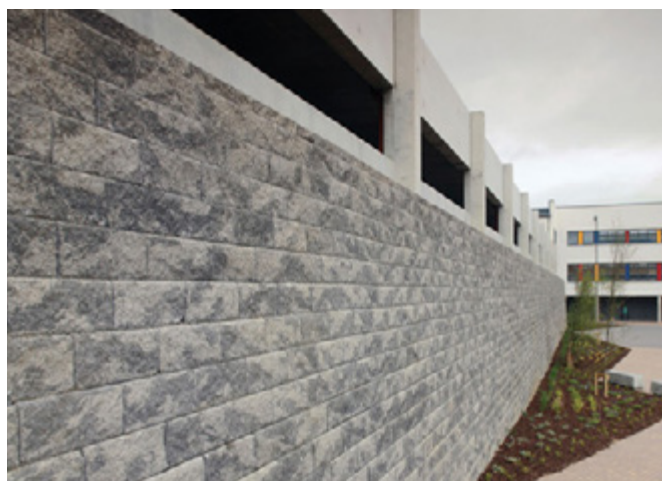
Close up of segmental MacWall® blockwork
