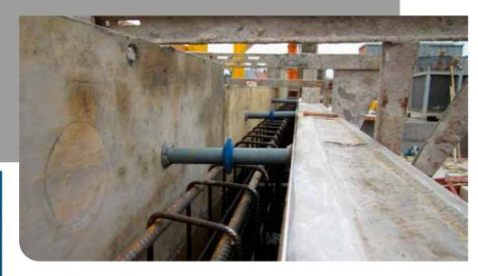
The Sealing UFO is designed to offer a more effective, quick and secure sealing solution than mastic or a length of water bar – both of which can be dislodged during the concrete pour.
