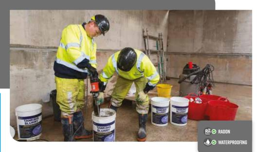
When mixed with clean water and applied correctly, this forms a permanent waterproof coating to the concrete and masonry and is easily applied by brush, roller or spray.
