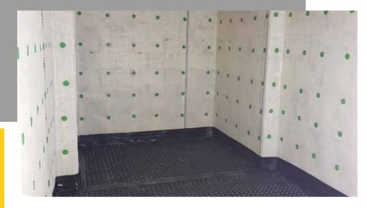
Wykamol **CM Plaster Plugs** and **CM Brick plugs** are of a high quality and can be used in a range of applications and on multiple substrate types. The tailor made Thermoplastic Elastomer seal ensures application of the membrane is water tight, if a normal fixing cannot be made then our **COB plugs** are ideal.
