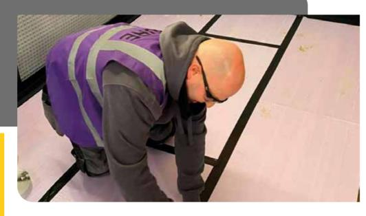
This high compressive strength material 500 KPa has a very impressive longterm compressive creep property of 225KN/m², meaning that even after 50 years the material will only compress by 2% if it is loaded at 225KN/m<sup>2</sup>.
