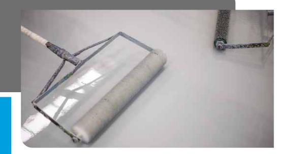
Epoxy sealer and surface damp-proofing membrane. **EP40 Finish Coat** is used in conjunction with **EP40 Primer**. **EP40 Floor Primer** penetrates the substrate, fills the pores and capillaries and improves the adhesion and evenness of the Finish Coat.
