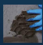
When mixed with clean water and applied correctly it is formulated for the rapid patching and plugging of active water leaks and seepagage in concrete and masonry.
