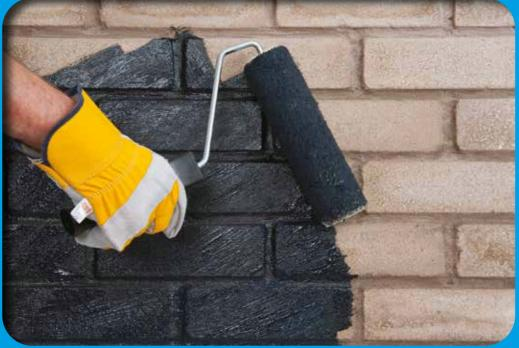
**External Type A Barrier Waterproofing**
