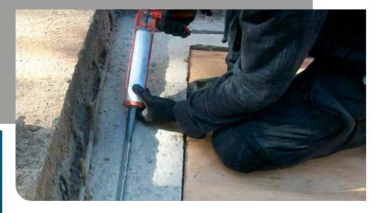
The hydrophilic properties of TT Swellmastic S2 display good consistency in swell rate during repeated wet/dry cycling. Expansion of the product on contact with water creates a positive pressure against the faces of the concrete joint, thus preventing the passage of water.
