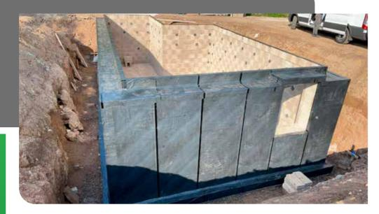
The high-density polyethylene film gives to the membrane characteristics of dimensional stability and ensures a uniform reaction to elongation stresses in a longitudinal and transversal direction.
