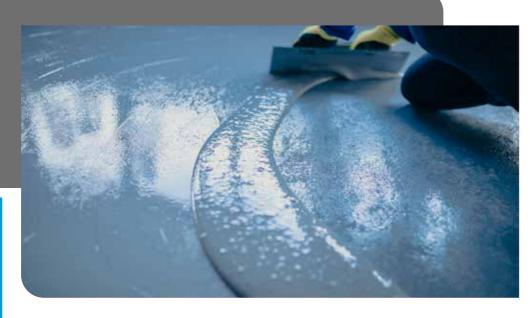
A solvent free, two-part epoxy resin coating primarily for use on screeded or concrete floors subject to rising damp or containing residual construction moisture.
