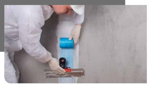
High performance joint and crack sealing system for joint and crack sealing for construction joints, expansion (movement) joints and connection joints or cracks.
