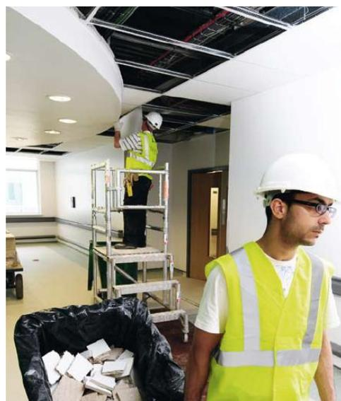
**Armstrong's recovery and recycling service:** segregation of mineral ceiling tile off-cuts at the point of installation.
