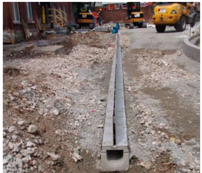
Installation of the solid slotted channel with grating in 4 mm stainless steel, with a neck dimension of 280 mm.
