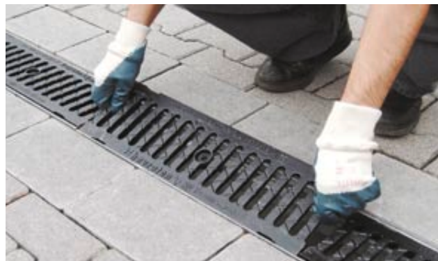
1. PUT SIDE-LOCK IN PLACE
