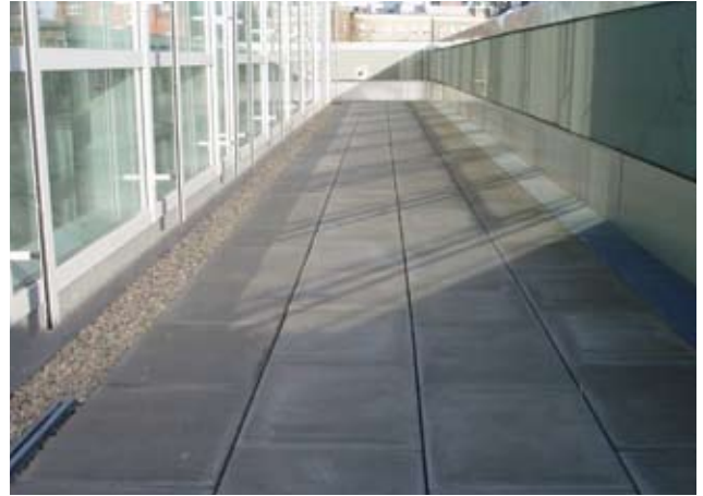
For draining the new roof terrace, a DACHFIX channel has been design specifically for this project.
