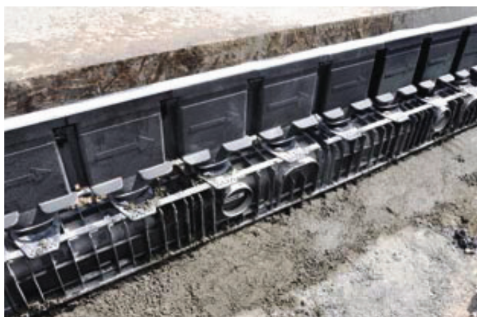
Channel installation at the new Formula 1 track, Yas Marina Circuit, Abu Dhabi
