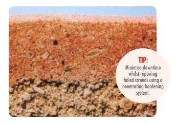
A penetrating hardening system (PHS), an epoxy material, is very versatile and ideal for fixing cracks, splits and flaws in a screed. It is applied over the top of the problem, soaks into the screed and hardens overnight, making it a very quick and effective solution.
