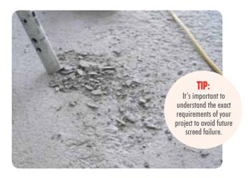
Too much liquid in the screed will also negatively affect vapour transmission control. If moisture vapour below the screed cannot evaporate out of the floor and gets trapped it will lead to unsightly blistering in the floor surface.
