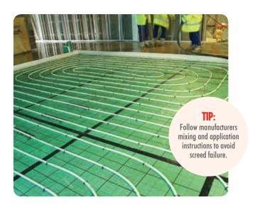
Project managers need to be careful when undertaking further work in an area with a floor that has insulation or underfloor heating. Point loading can put too much pressure into one area which can collapse the insulation, creating a weak point where the screed could cave in if the stress continues. A common example of this is when cherry pickers are positioned on the floor and the heavy, continual stress under the feet puts too much strain on the insulation and screed.
