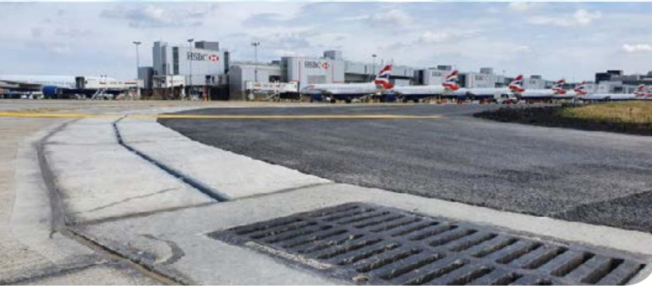
In some projects there may be a requirement to install the slot drain system to follow a given radius, for example around the perimeter of a taxi-way on an airport project, or following the curve of a landscape feature.
