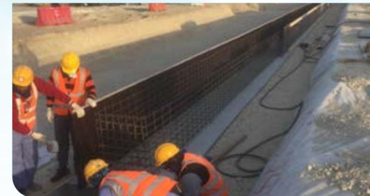
Fitting of the steel reinforcement cage can be carried out away from the trench, making the task easier for the contractor. The completed unit can then be lifted into the trench.
