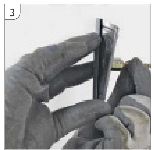
At downpipe joints, mark positions for the v-locks at every 2 metres (maximum). Then firmly screw-fix the v-lock to the wall.
