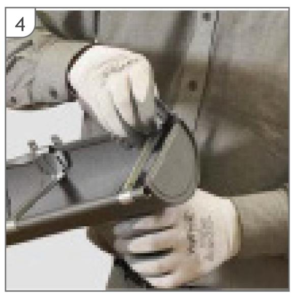
Always use two concealed brackets to secure the running outlet.
