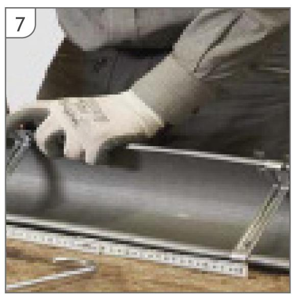
Clip concealed brackets to the cut lengths of gutter at 400mm max centres.
