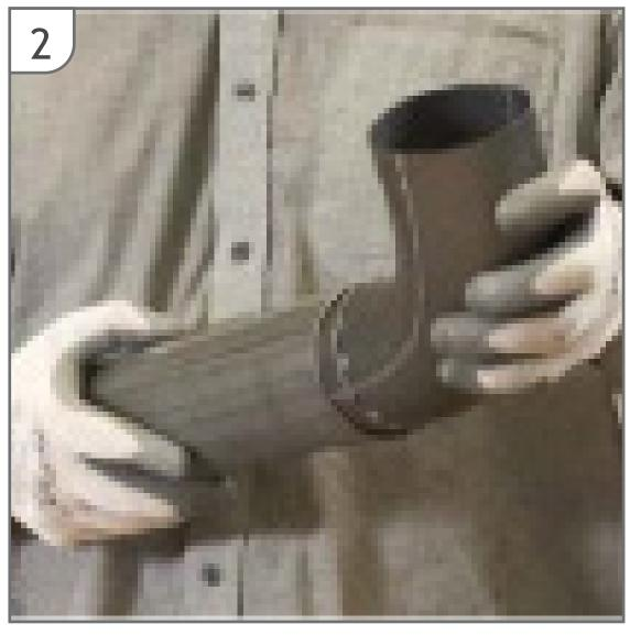
Once measured, fit the two bends together. It may be necessary to extend the assembly using a piece of downpipe.
