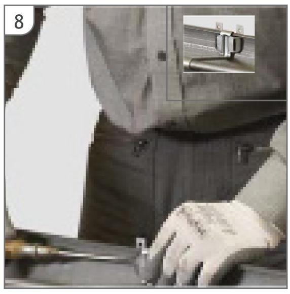
Secure each bracket to the gutter by folding in the two tabs. Then thoroughly clean the gutter joints before gluing.
