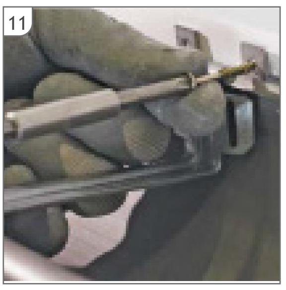
Fix the gutter brackets according to the chalkline.
