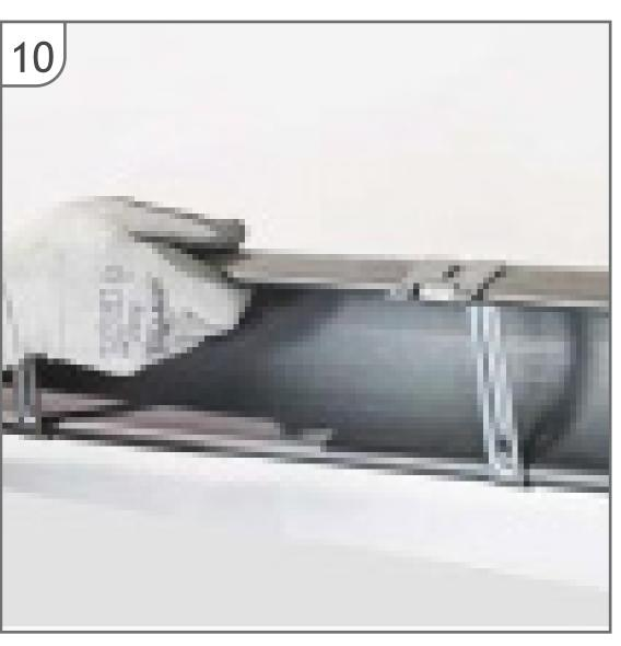
• Insert the prepared gutter into the already installed running outlet via the rolled front edge first. Ensure a 50mm min overlap. Pliers can be used to ease open the beading on installed gutter.
