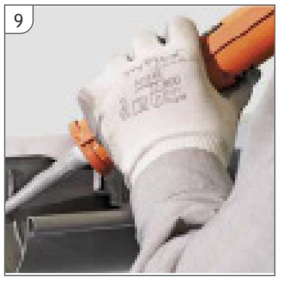
Apply two, thin, parallel beads of Quartz Zinc adhesive to the inner surface of the running outlet at max 50mm from the edge.
