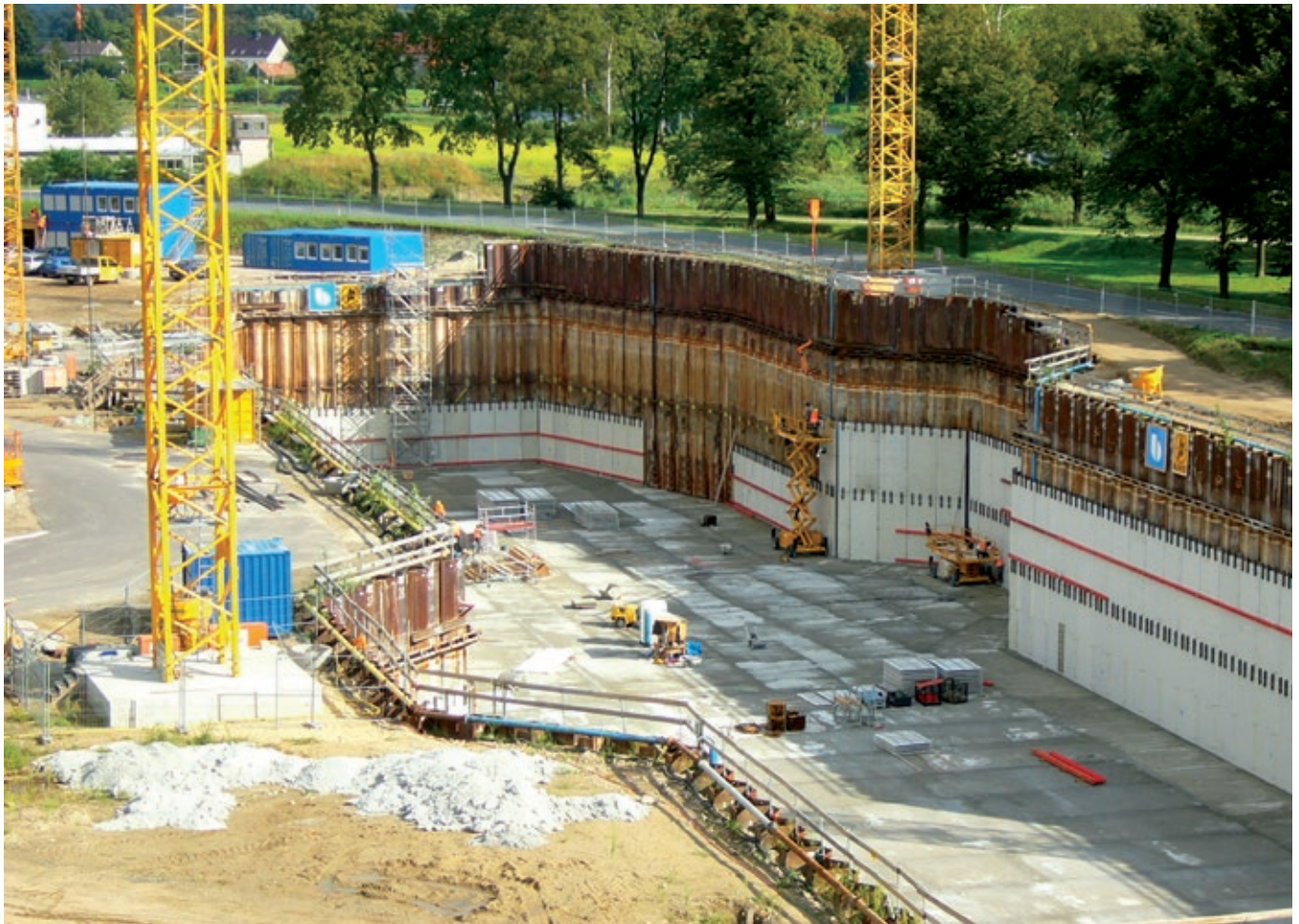
Our reference in Niederfinow (Germany): Boat lift's fundaments
