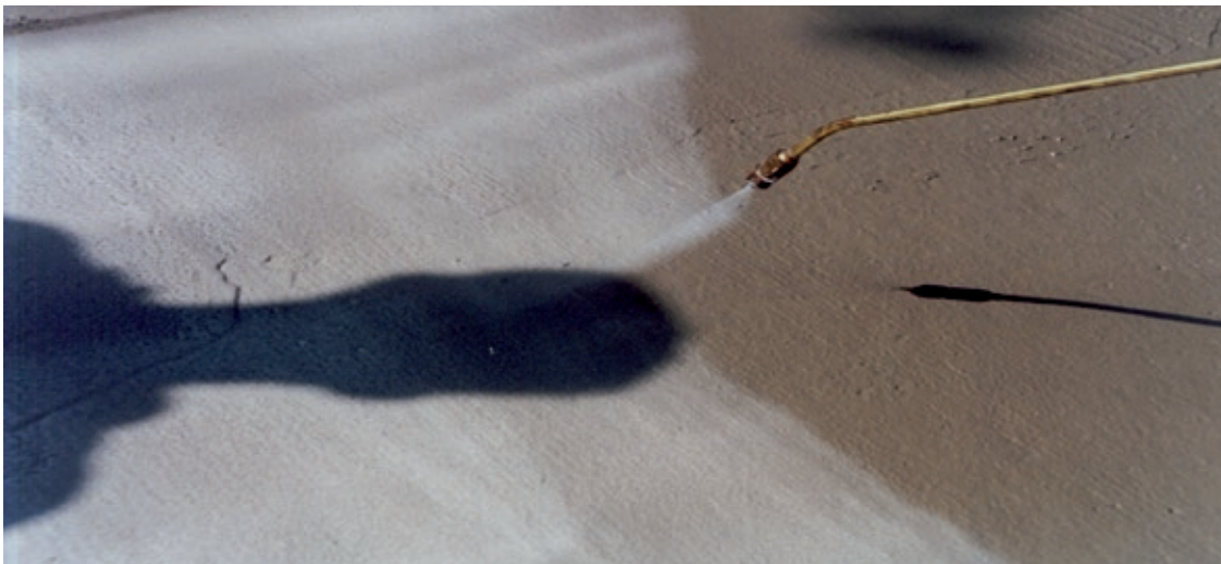
MasterKure application on construction site after placing the concrete
