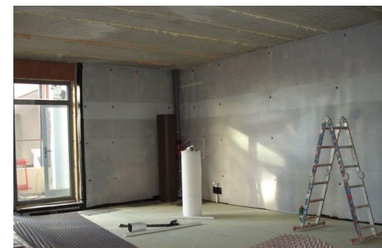
Newton cavity drain membranes applied to the walls
