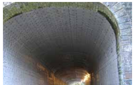
Newton 508 Mesh being applied to the walls
