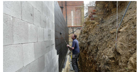
Newton 902 Primer applied prior to 410 membrane
