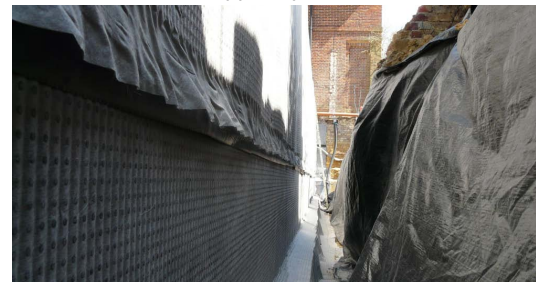
Newton 410 Geodrain applied prior to back fill
