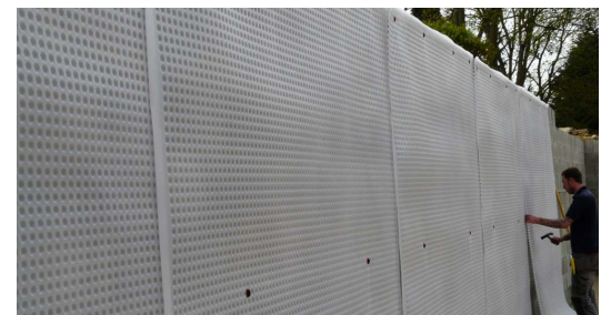
Newton System 500 being applied to the internal blockwork
