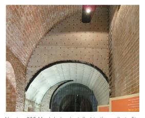
Newton 503 Mesh being installed to the walls to fit the contours of the structure
