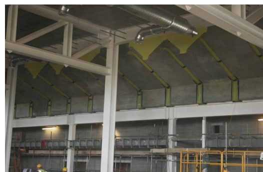
Newton 503 and 902 applied to the underside of the grandstand construction joints
