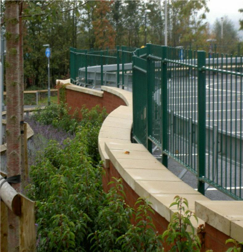
Copings designed to compliment brick walling to external works of large retail park development. Supply of non-standard coping units for all external walling to all boundary walls, car parking area, retaining walls and stairways including radiused units and provision for railings.
