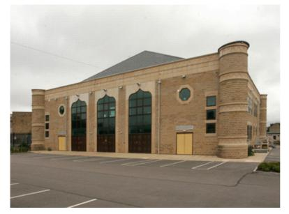
Non-standard stone units to complement natural stone walling to clients specification. Non-standard units individually designed in conjunction with client and architect.
