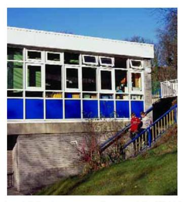
Dilapidated timber at St Mary's Church of England Primary School in Dover, Kent has been replaced with Celuform 150mm white shiplap PVC-ue cladding. The cladding creates a low maintenance deep fascia around the perimeter of the school buildings.
