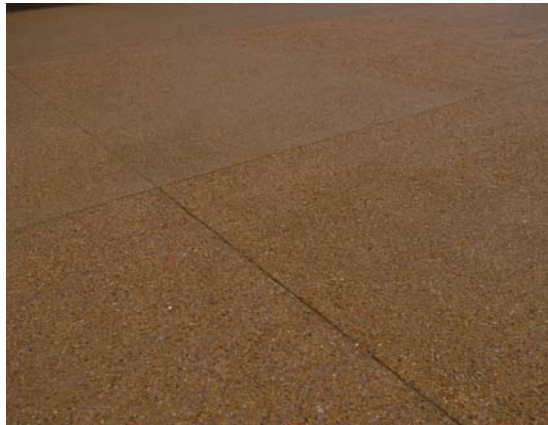
Paving with exposed aggregate finish achieved by VBA Surface Retarder
