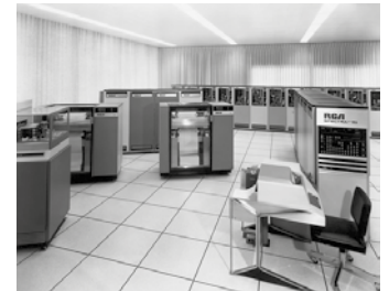
One of our early access flooring installations, from the 1960s.
