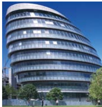
The Greater London Authority offices – one of many prestigious buildings where John Beckett installed Kingspan flooring.
