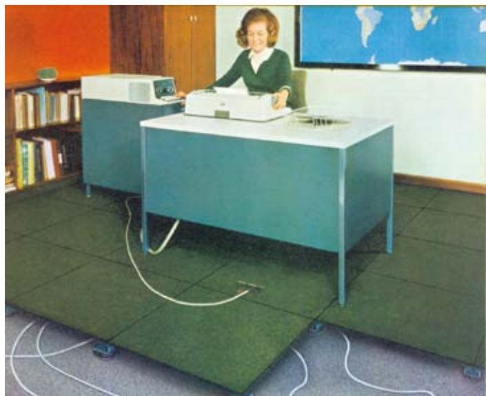
A RAM flooring installation in 1970.
