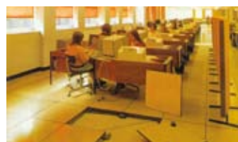
RAM flooring installed at Empire Stores Ltd in Bradford in the early 1970s.
