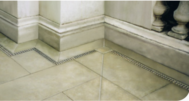
Custom made gratings Cast iron grating and show edge coupled with stainless steel channel provided a complete drainage solution to blend with the period architecture at Somerset House, City of Westminster.
